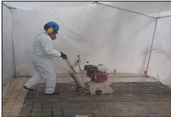
Old tile removed and concrete scarification.
