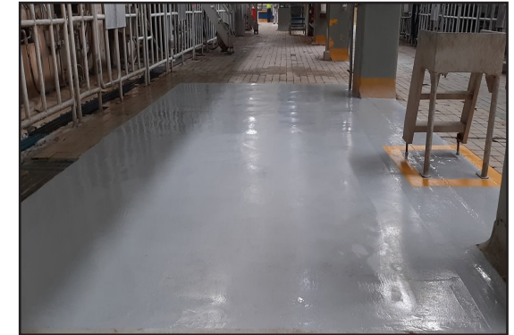
ARC S2 with broadcast and sealer coat.
