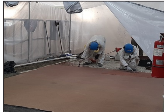
Resurfacing with ARC EG-1.
